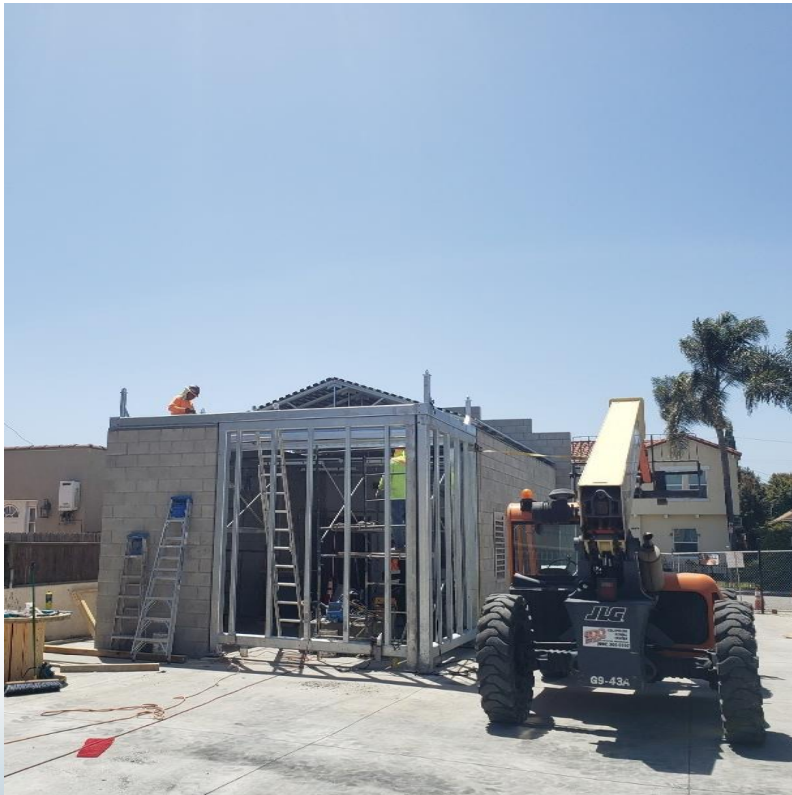
Framing & Metal Roof Panels
