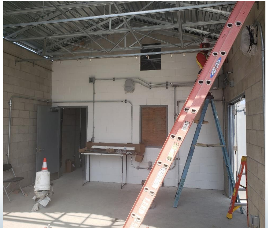
Framing & Metal Roof Panels
